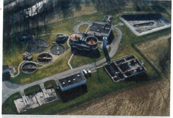
Photo of a modern sewer treatment plant
