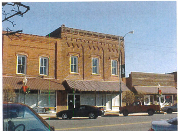
Traditional construction in small town commercial areas within the central Piedmont region.
