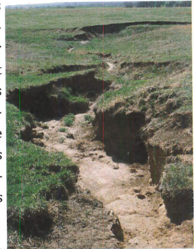
An erosion gully in a pasture.
